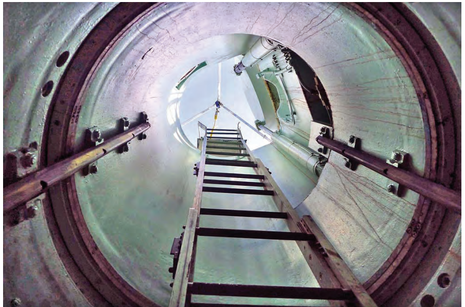
A view up the personnel access shaft at D-9 LF
